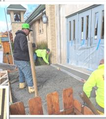
Two steps with handrails on both sides were added at the sidewalk to assist people up to the entry, increasing safety for all.
